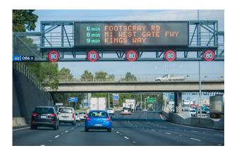
Road authorities around Australia have been using Transmax's smart motorways technology since the late 1980s. It all started with a traffic management system being installed in Brisbane, Queensland with features including ramp metering, graphical displays of traffic conditions, and automatic incident detection.
